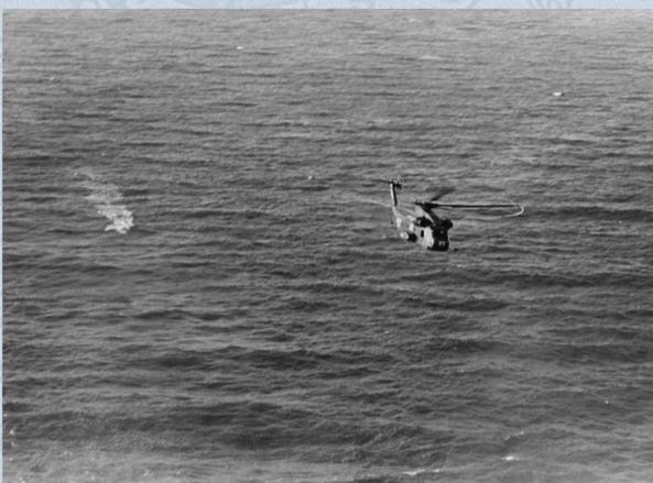
*Operation END SWEEP. A CH-53A Sea Stallion tows a Magnetic Orange Pipe (MOP) to detect mines for clearing Haiphong Harbor. To reduce collateral damage after U.S. demands were met in peace negotiations, U.S. Navy ships and aircraft cleared Vietnamese waters of mines. (U.S. Navy / National Archives)*
